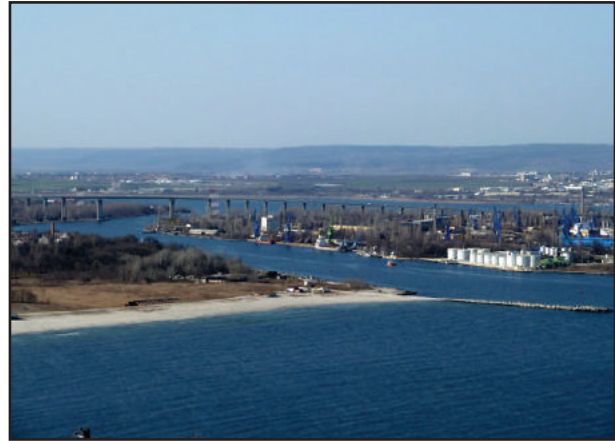
Fig. 5 The deep-water navigational channel (Varna Bay)
