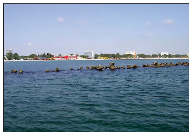
Fig. 7 Breakwater (Mamaia resort)
