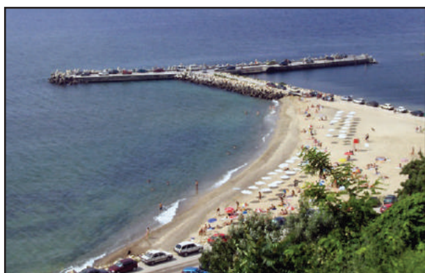
Fig. 2 “Groyne” with port and coast-protection functions
